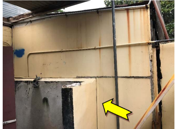
Photo 2. Interior, throughout, walls - suspected lead-containing cream upper paint system.
